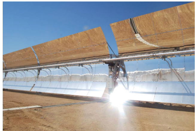
Figure 3: Solar Thermo-electric Plant in Puertollano (50 MW); Investment: M€28; Estimated Net Production: 41GWh/y
