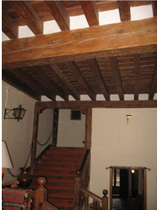
Fig. 3.- Aspect of the underside of the forged of duckboard of la casona del siglo XVII used as an example in this section.
