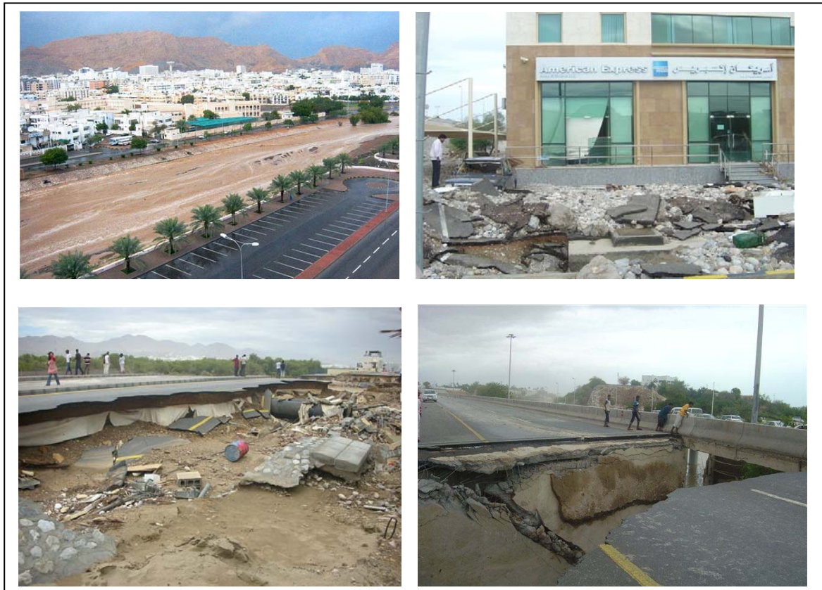
Figure10: Destructive effects of storm floods at Muscat (CAE, 2007)
